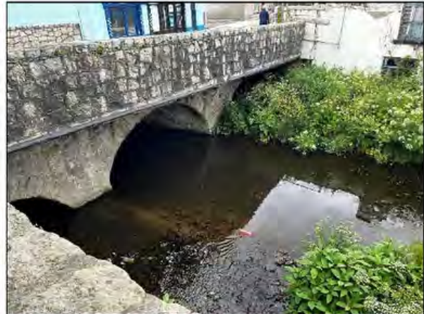
Photo 4: Downstream Bridge Openings
