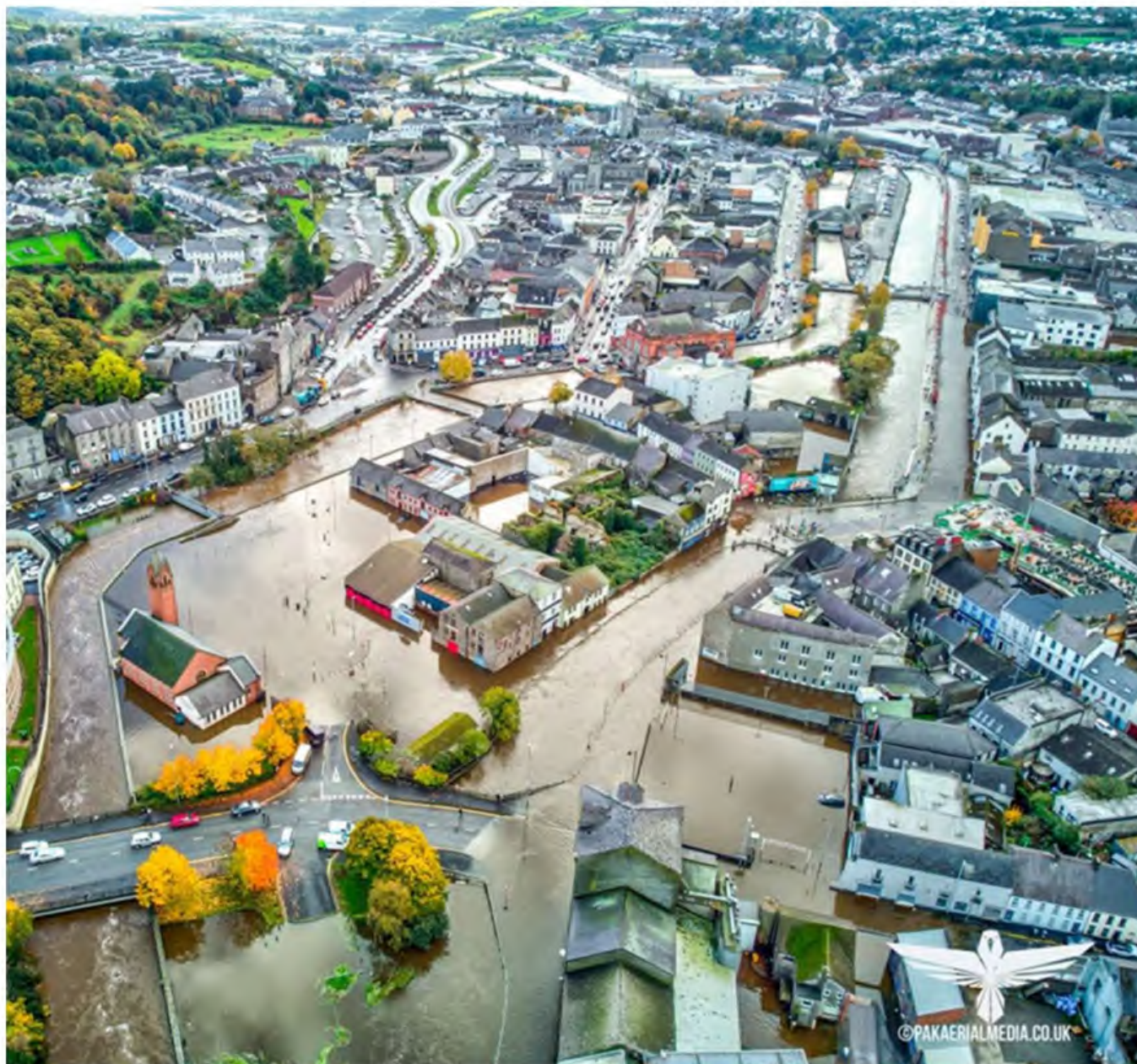
Aerial Photo of Flooding in Newry 2023
