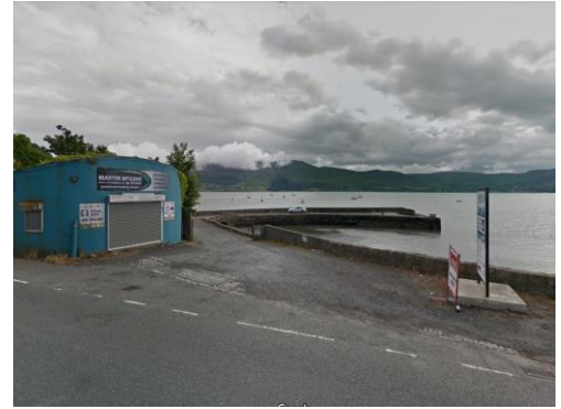
The pier opposite JC Campbell on the Shore Road
