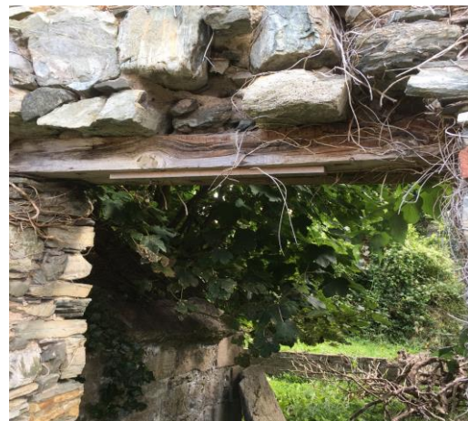
Closeup of a wooden beam which is supporting the belltower
