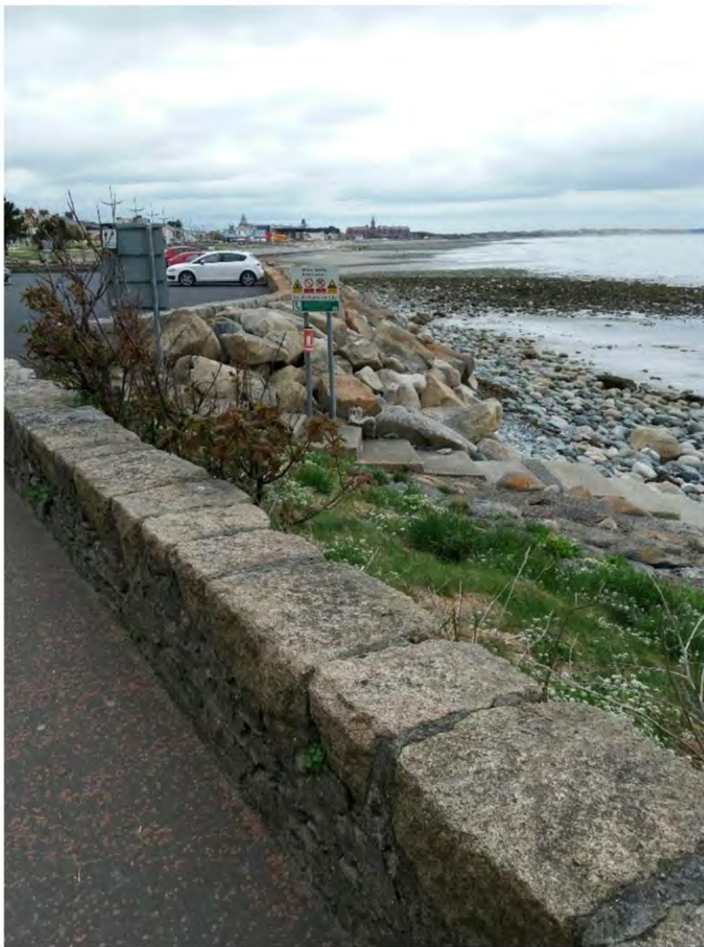
Photo 1 - View of steps and adjoining car park
