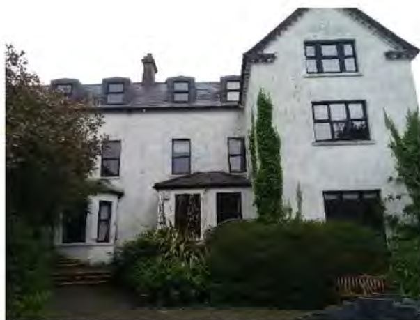
Existing building - wing to be demolished
