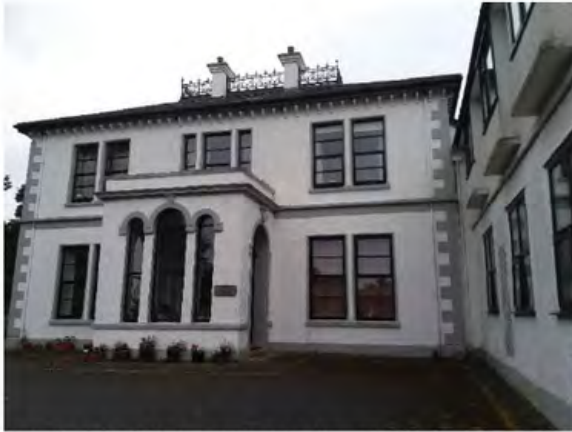
Existing building – wing to be retained
