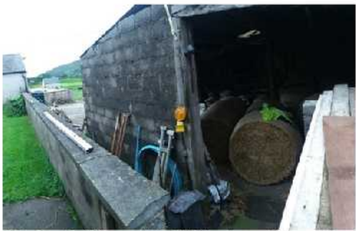
Existing buildings at No.73 Newtown Rd
