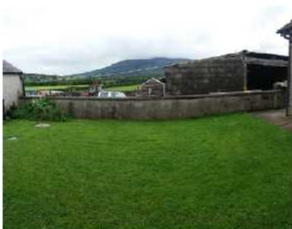
Existing buildings at No.73 Newtown Rd
