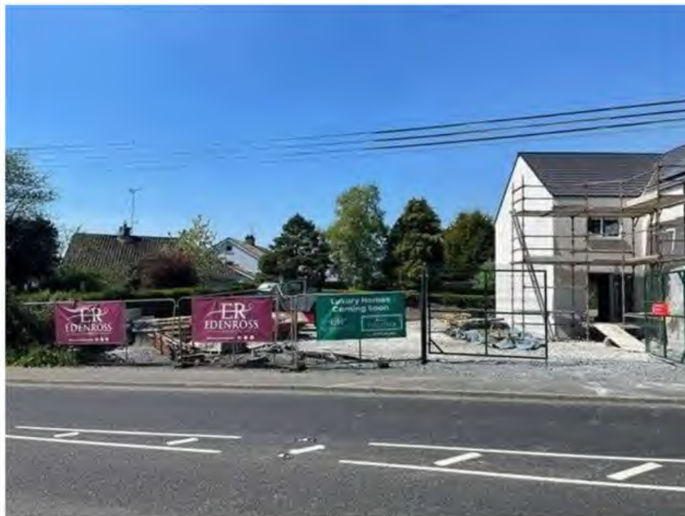
Figure 2- Application Site Viewed From Rathfriland Road
