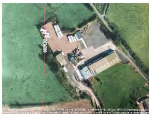
Site including area of unauthorised works
