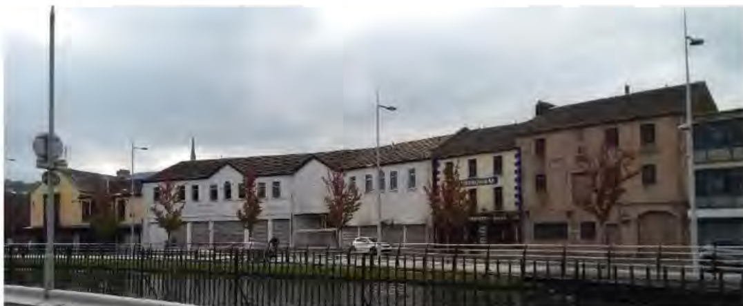
No's 49-54 Merchant's Quay (white building.)
