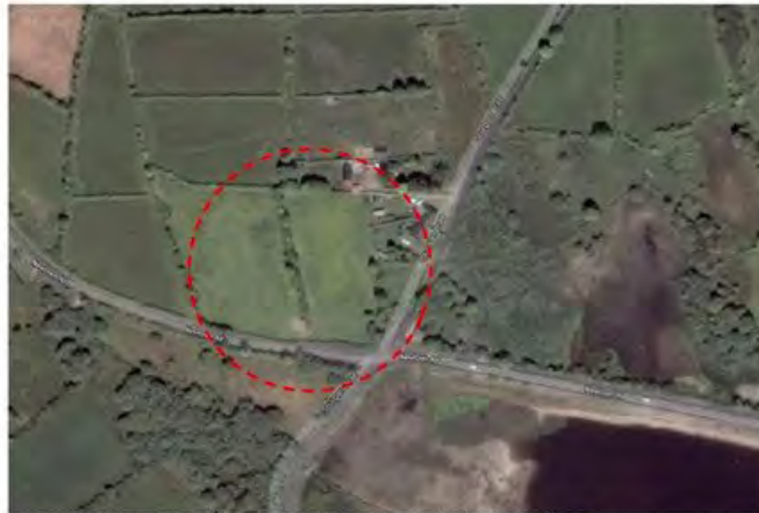
Site overview showing adjoining existing dwellings and agricultural buildings
