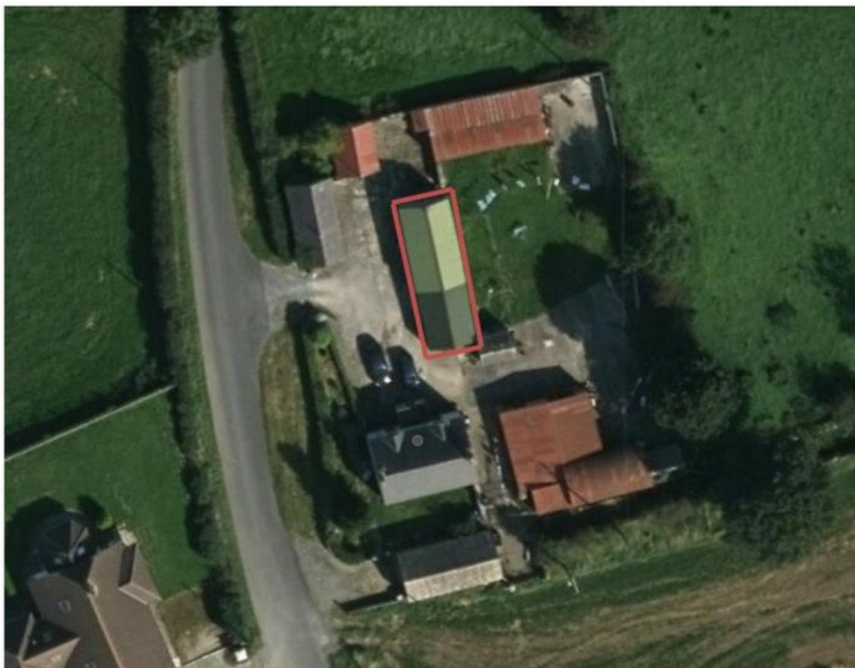
Subject building outlined in red
