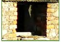
Formerly part of a built cluster, the structure is typically vernacular of the mid-1800s – load bearing mass rubble walls bonded with lime mortar - intact and sound – harled externally – lime
