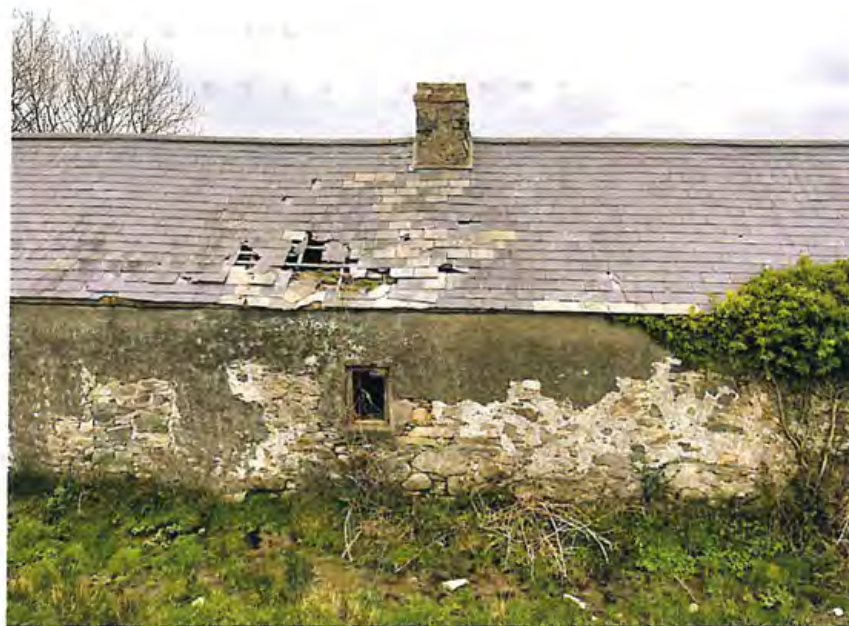
Figure 4.0 Localised loss of slates on rear slope
