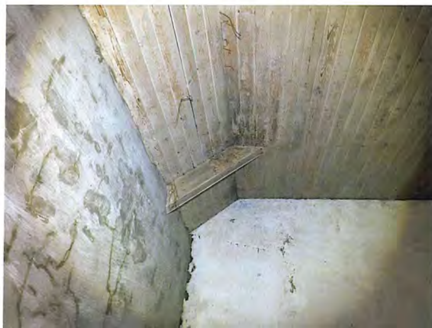
Figure 13.0 Visually sound truss end and ceiling
