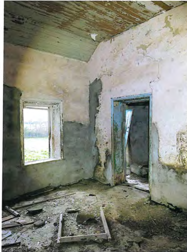
Figure 12.0 Cracks associated with timber lintels
