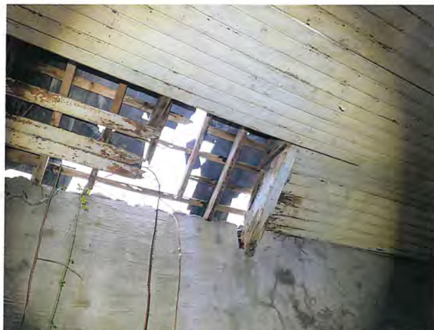
Figure 14.0 Failed truss end and rafter tails
