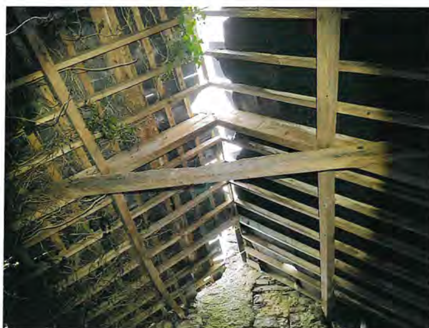
Figure 3.0 Timber roof over byre
