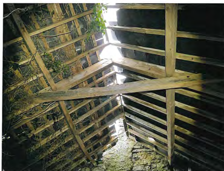
Figure 15.0 Byre roof damage
