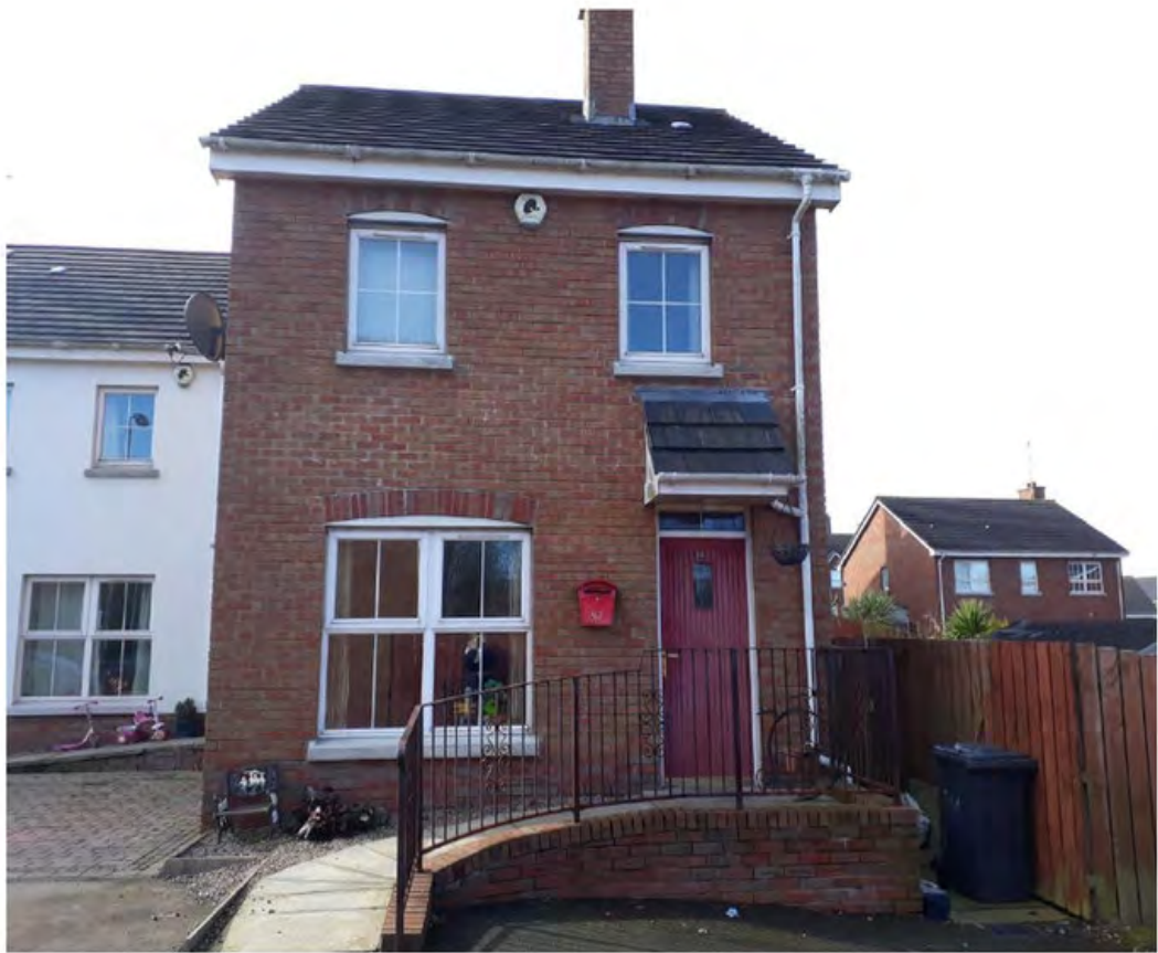
Front elevation of 36 Demesne Heights
