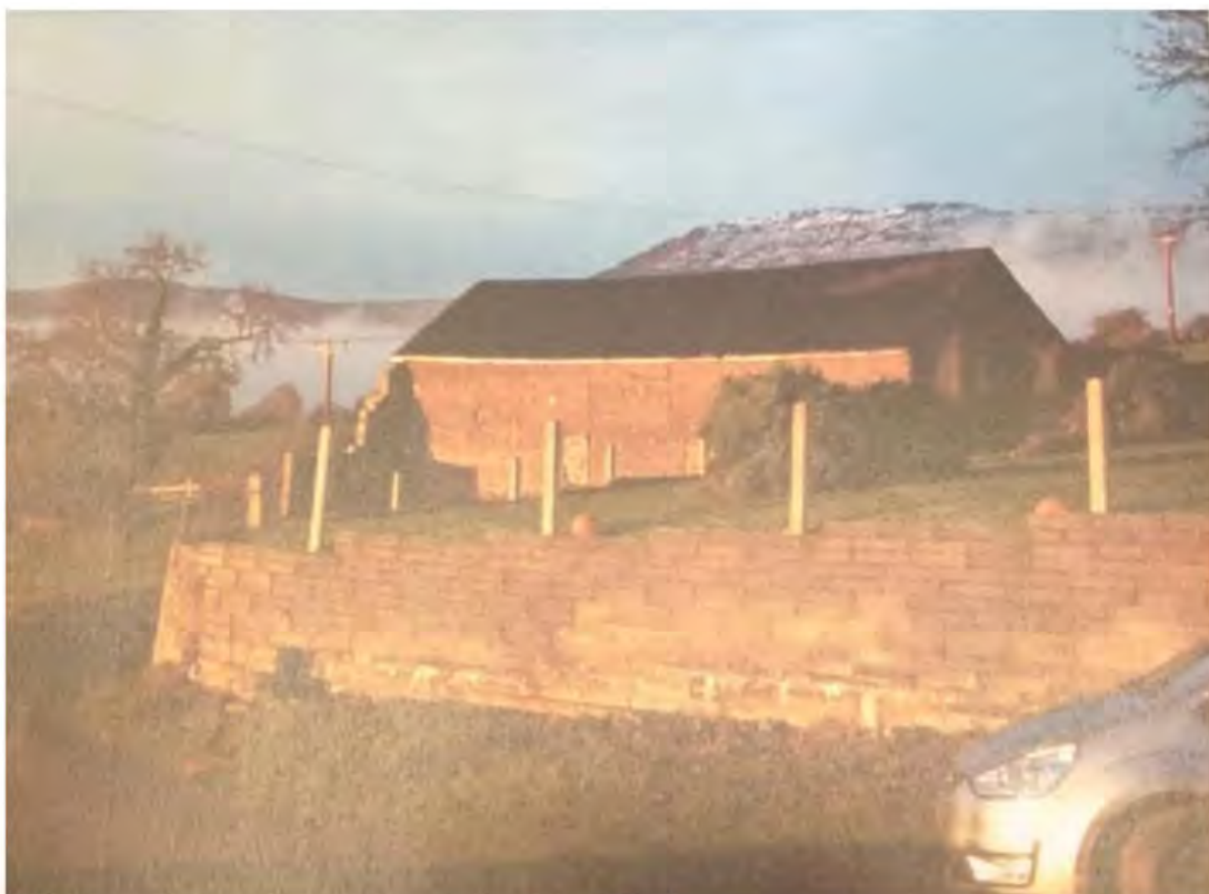
Objectors photograph – view towards original shed
