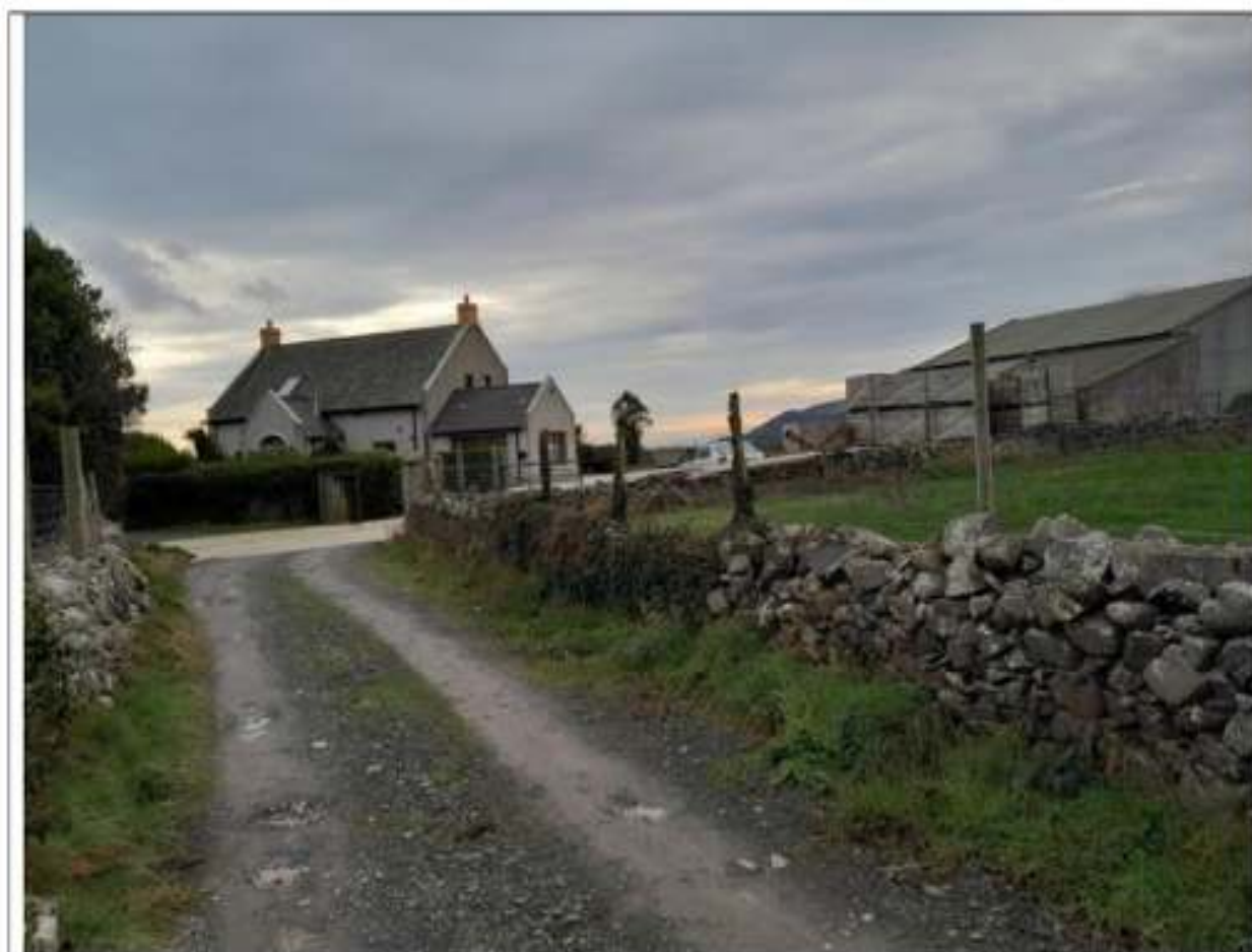
Dwelling and sheds at no. 51 with application site in foreground
