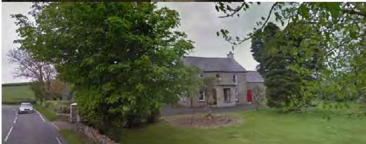
View from google street
