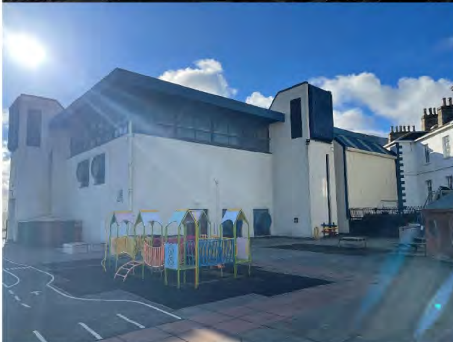
Rear Extension Proposed for demolition
