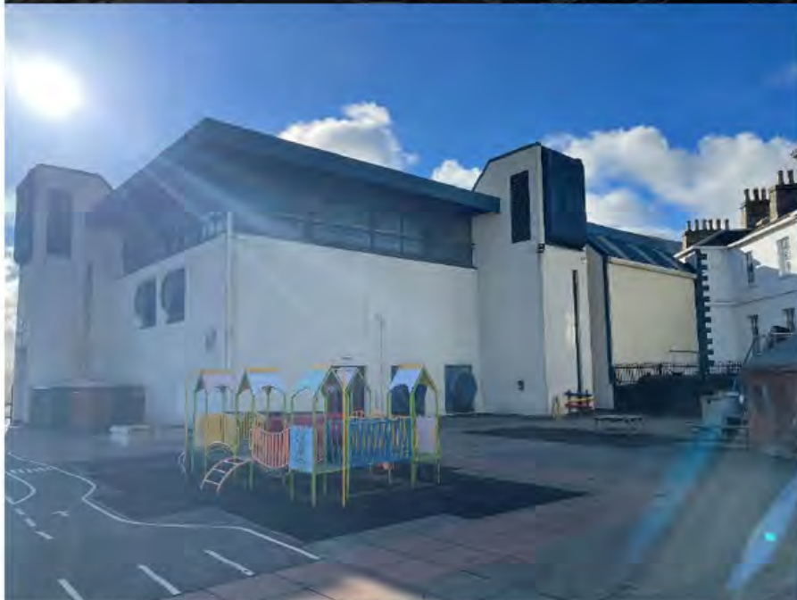
Rear Extension Proposed for demolition
