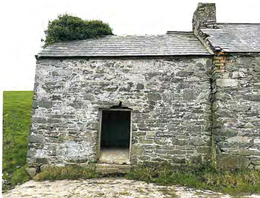
Figure 8.0 Byre door opening
