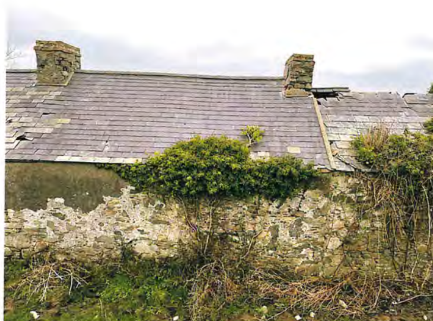
Figure 5.0 Central and south chimneys
