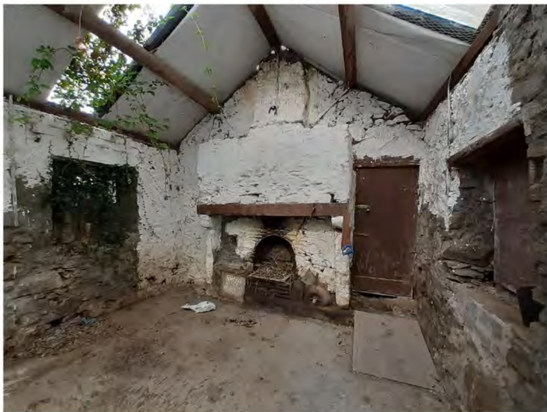
Internal view of building to be replaced
