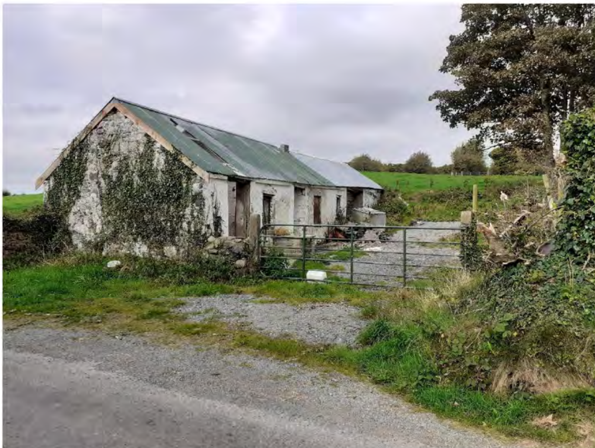
Building to be replaced
