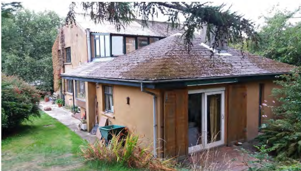
Single storey building to be replaced
