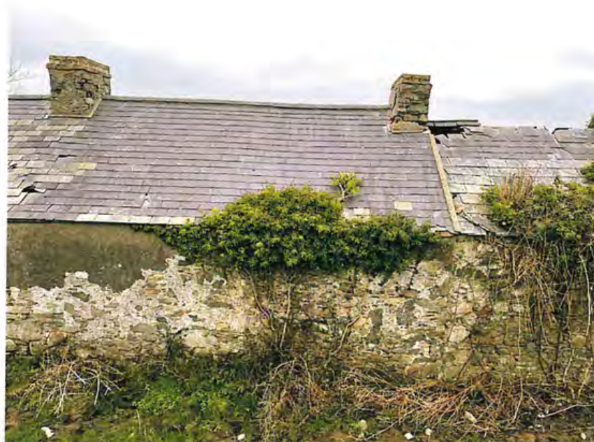
Figure 5.0 Central and south chimneys
