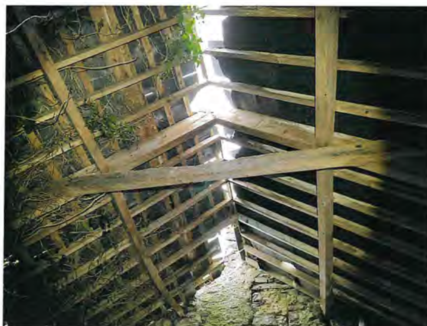
Figure 3.0 Timber roof over byre
