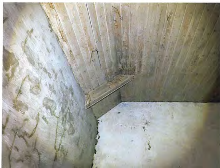
Figure 13.0 Visually sound truss end and ceiling
