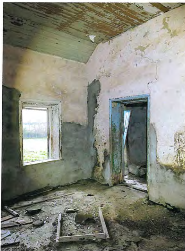
Figure 12.0 Cracks associated with timber lintels
