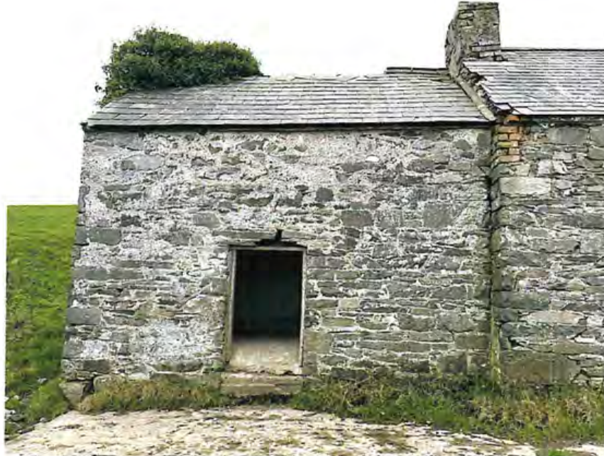
Figure 8.0 Byre door opening
