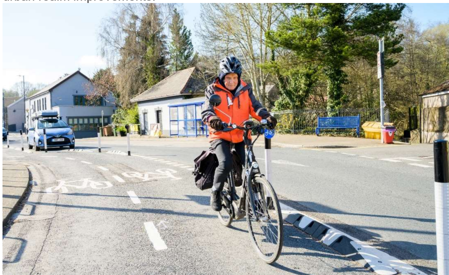
Cycle track constructed using temporary materials
