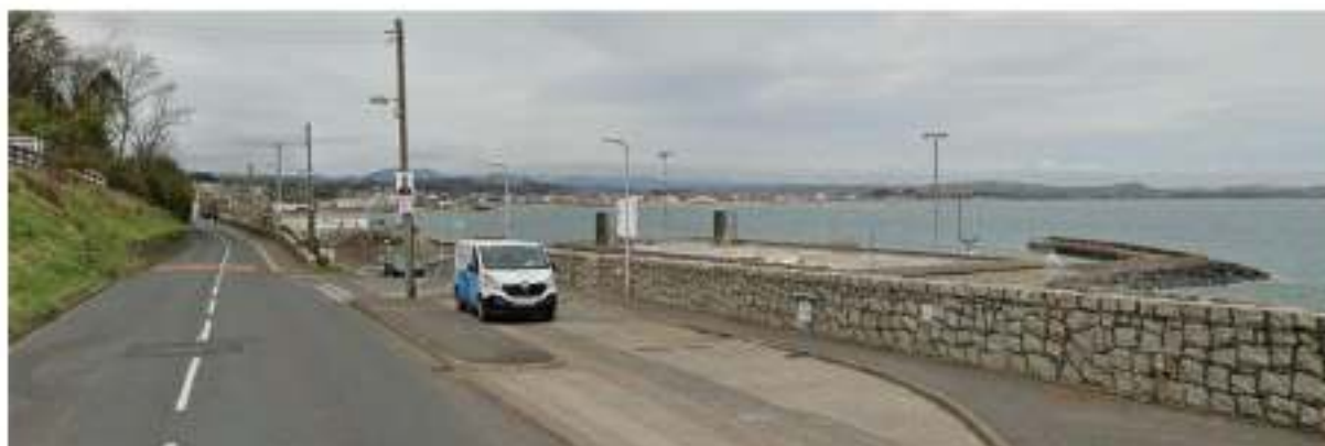
Entrance off Kilkeel Road to South Pier of Newcastle Harbour
