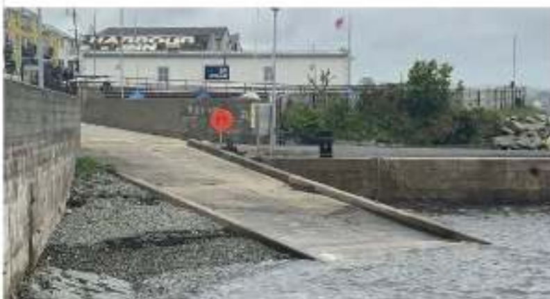
Figure 5 - Slipway located immediately south of north quay.
