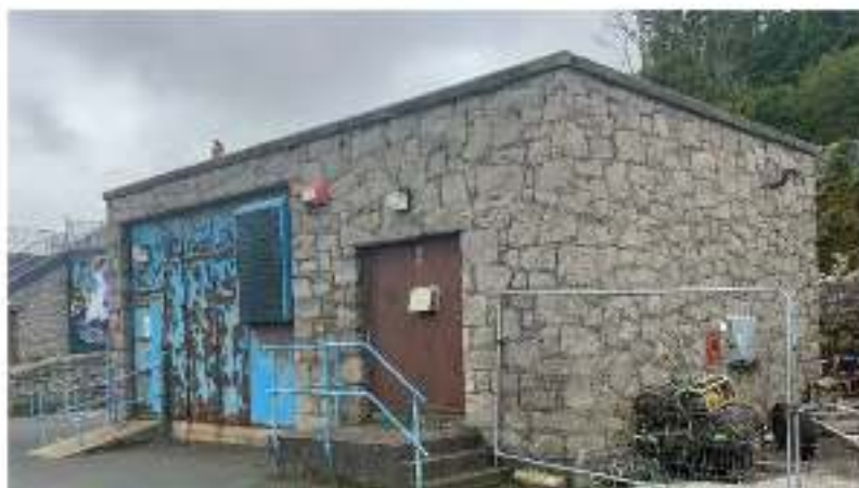
Figure 9 - Former pump house from northeast.
