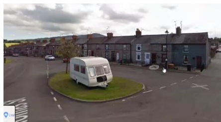
The area requiring resurfacing
