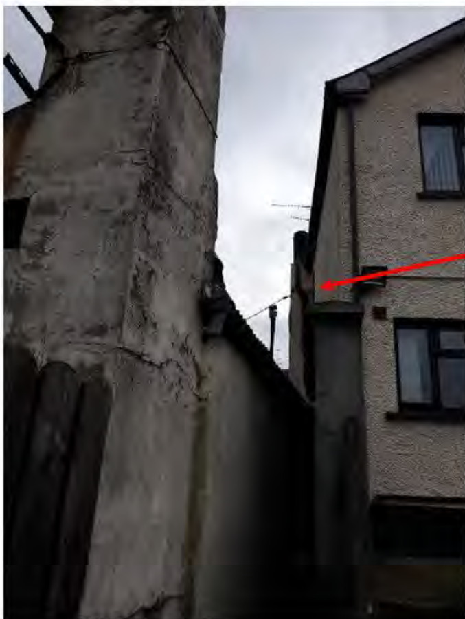
Position of bathroom window, no 56
