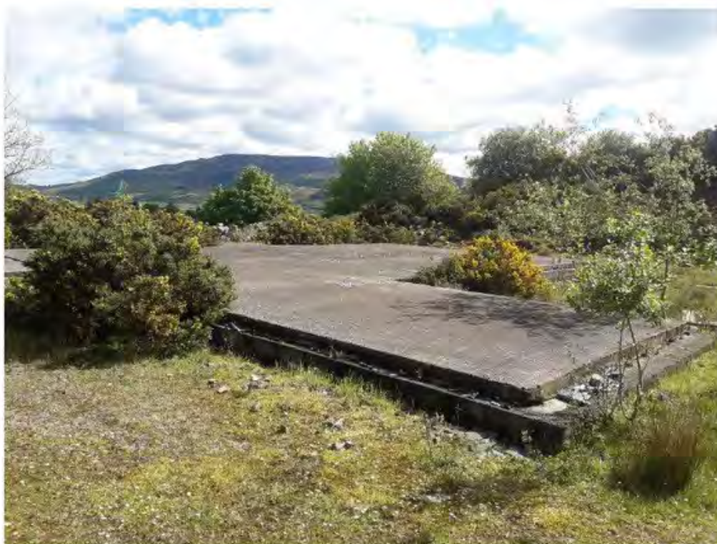
Looking north onto existing foundations
