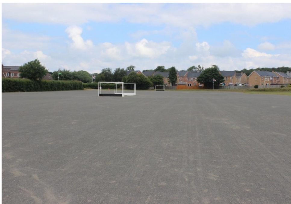
The two shale pitches at Langley Road Playing Fields, both in good condition but no longer accepted by Hockey's governing body for hockey at any level; one pitch has floodlights (8 no.).
