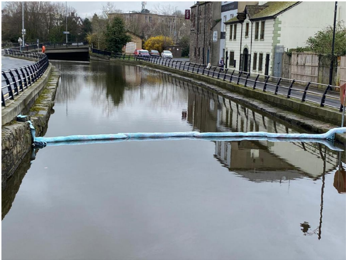
Booms placed to prevent oil spreading along canal towards City Centre
