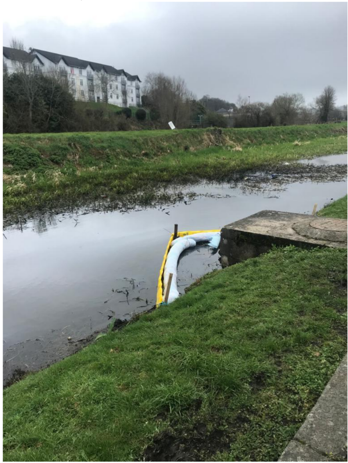
Boom at source of oil spill
