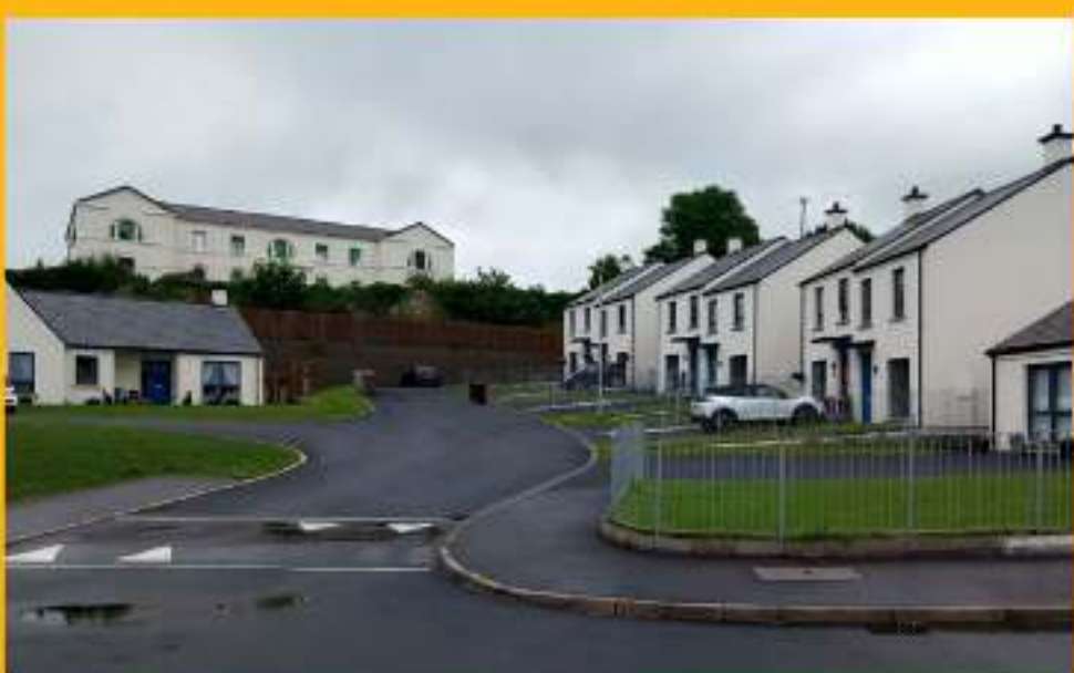
Downs Hospital, Down public scheme (Cairn HA) which is currently on-site.
