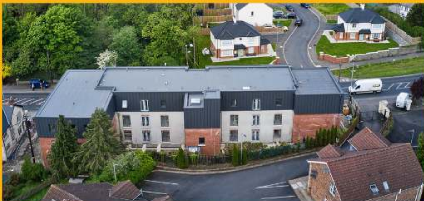
Belfast Road, Newry scheme (Arbour Housing Association) which has recently completed
