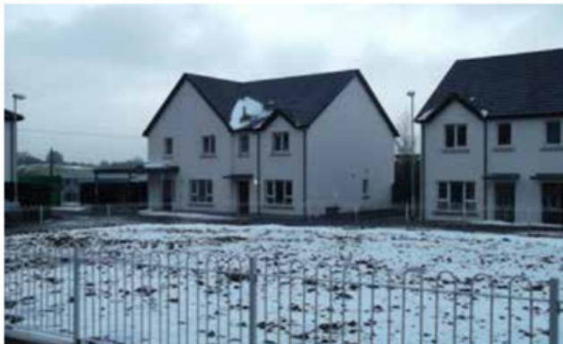
Social Housing at Millvale Road, Bessbrook (Apex Housing Association)
