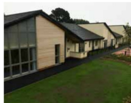
Supported Housing scheme at Newry St., Killeel (Choice Housing Association)
