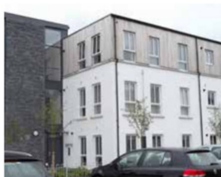
Social Housing at Ballynahinch (Choice Housing Association)
