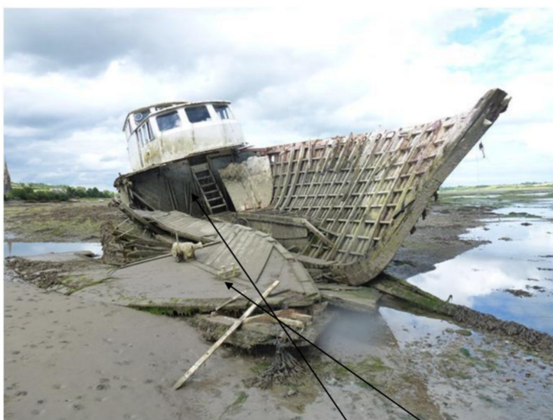
No.4 photo showing forward section of starboard side hull planking missing. Fore deck in one piece broken away from vessel. Bulkhead division into engine compartment
