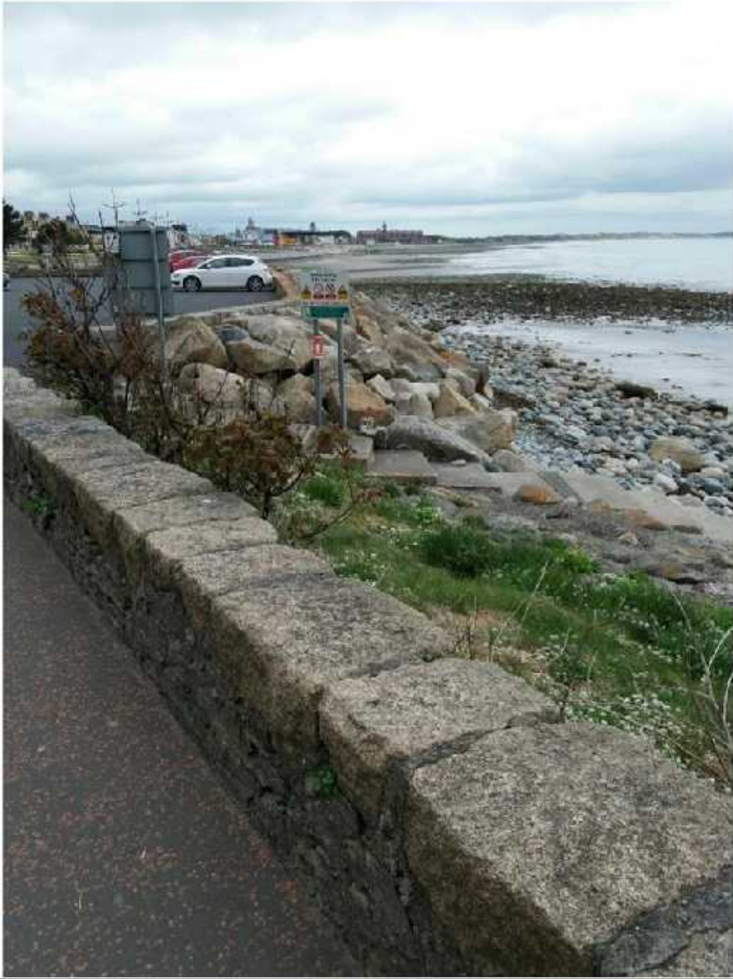
Photo 1 - View of steps and adjoining car park
