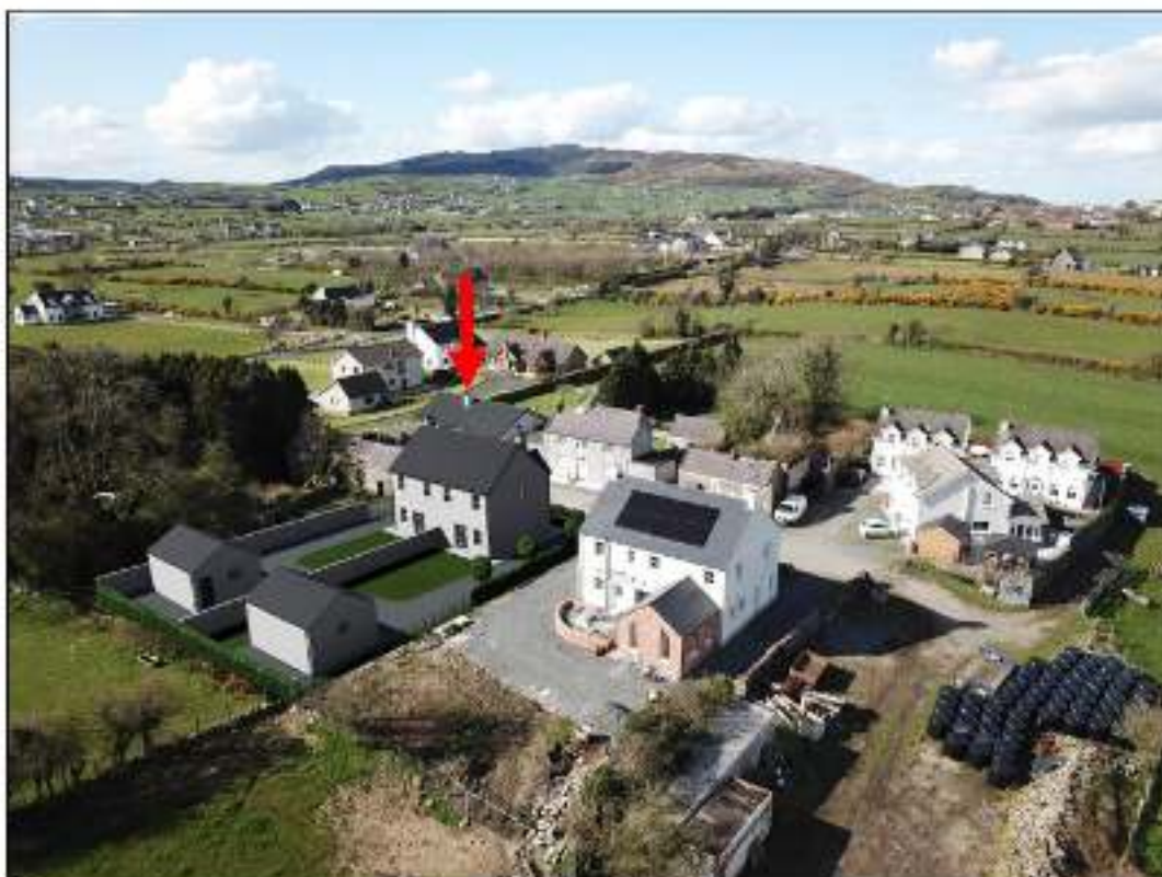
1E) View looking North East at the Proposed dwellinghouses and the existing pattern of development along the Newtown Road.
