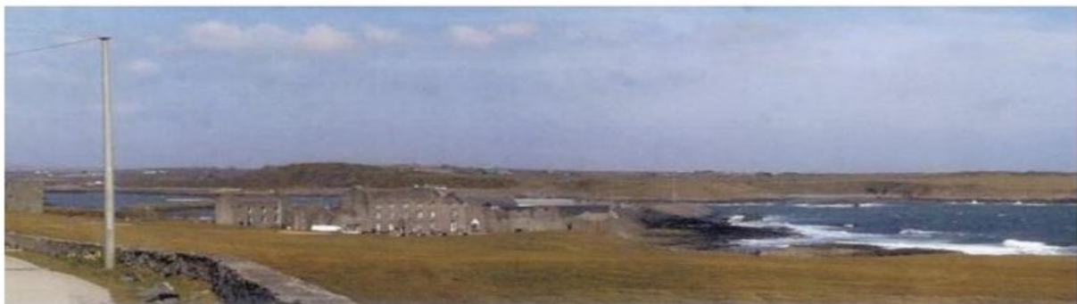
Existing View from Castle Place Ardglass
