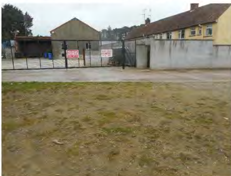
Photo 4 – Maintenance shed backing onto Austin Terrace
