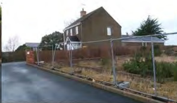
No 12 – adjacent and west of the site
