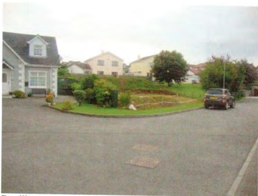
Dwelling to rear of No. 1 Whinnbloom and adjacent site to rear of No. 2 Whinnbloom (foundations)
