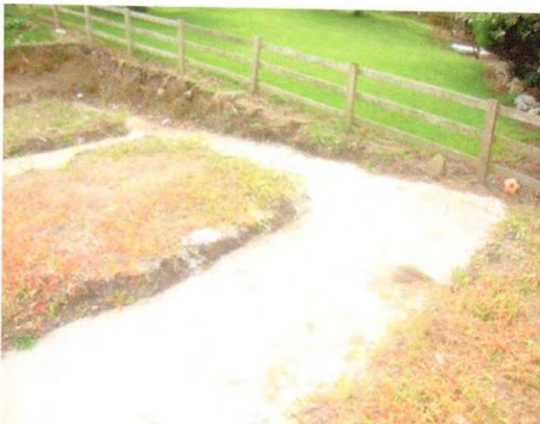
Level difference can be accommodated by minimal cutting as demonstrated by foundations of part built property to the north.
