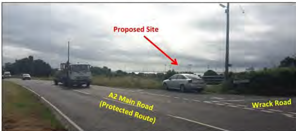
Image 1 - View of the Application Site
