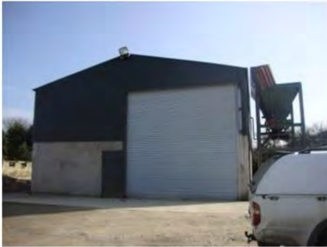
Existing shed to be retained
