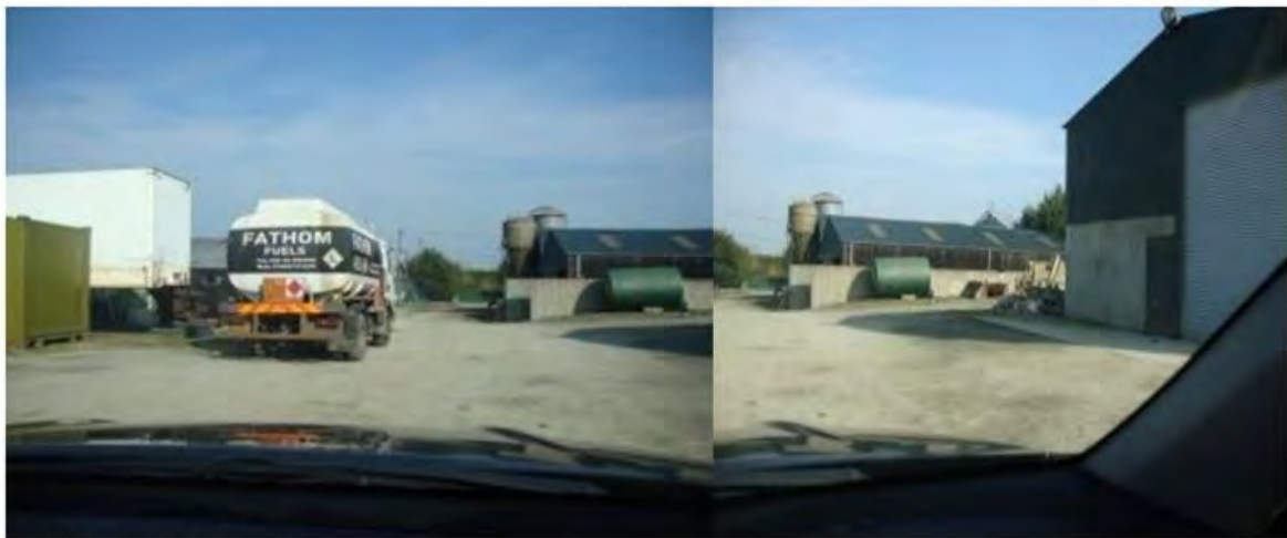
Existing yard and shed
