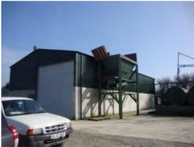
Existing shed to be retained
