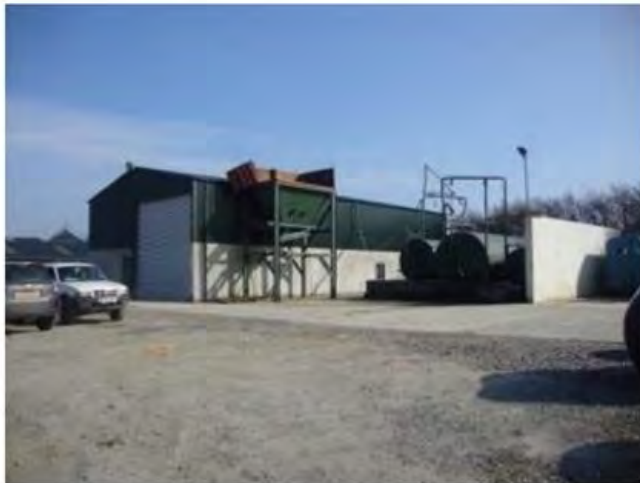
Existing shed and yard to be retained
