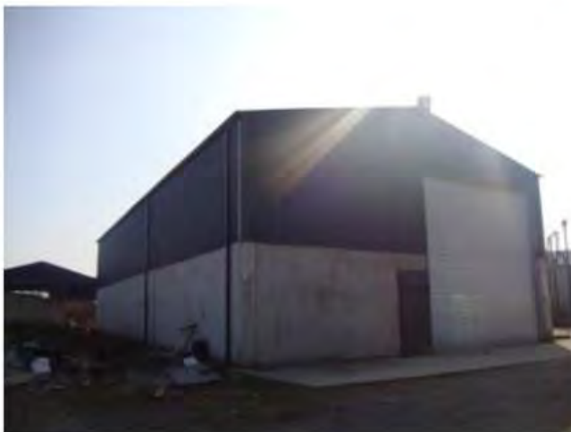
Existing shed to be retained
