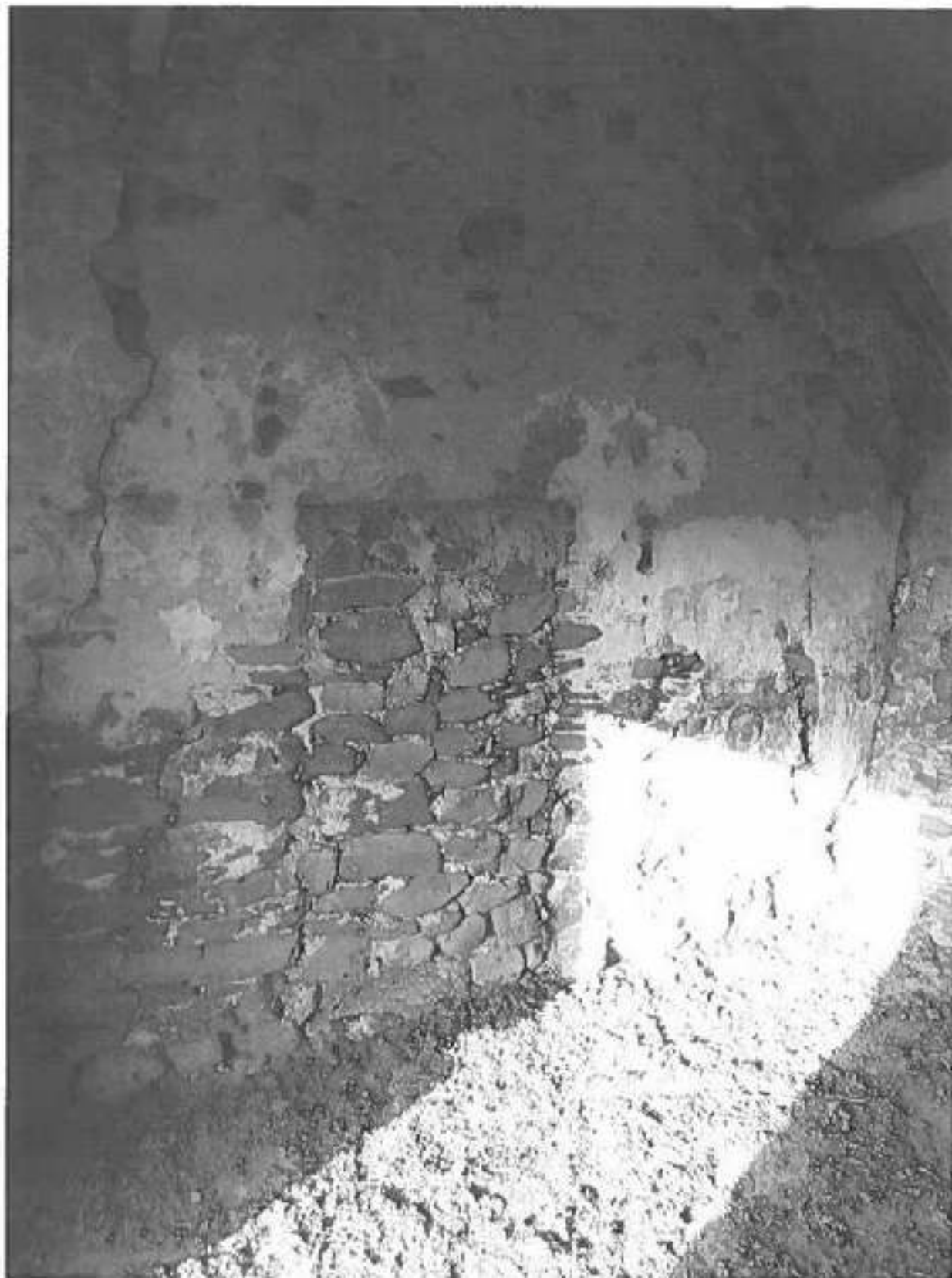
Plate 2: Evidence of the blocking up of an internal doorway.
