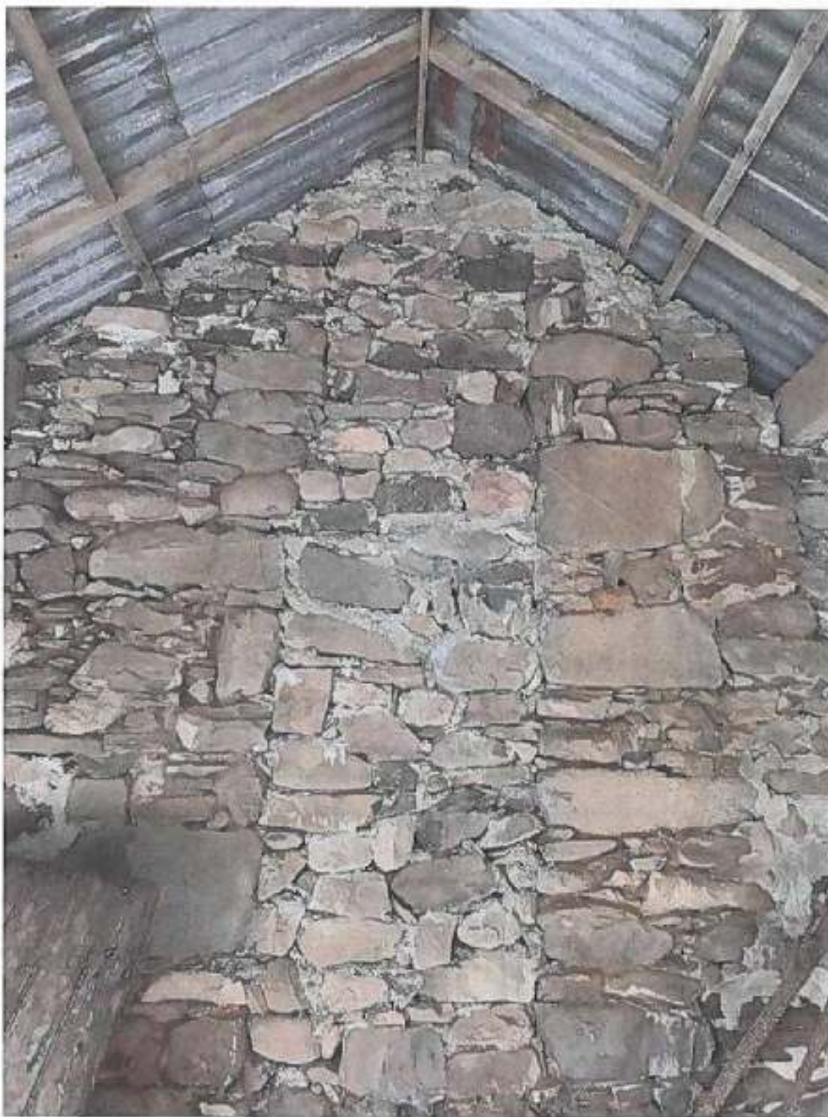
Plate 3: Evidence of the blocking up of the former fireplace/chimney.
