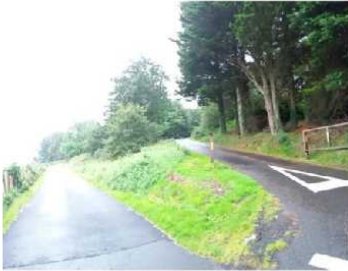
North of embankment looking South
