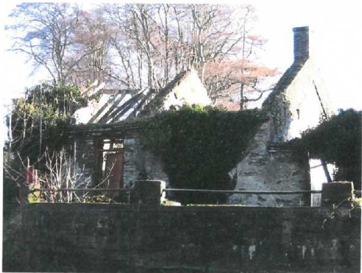
Existing Dwelling LHS Frontage to Vianstown Road.
