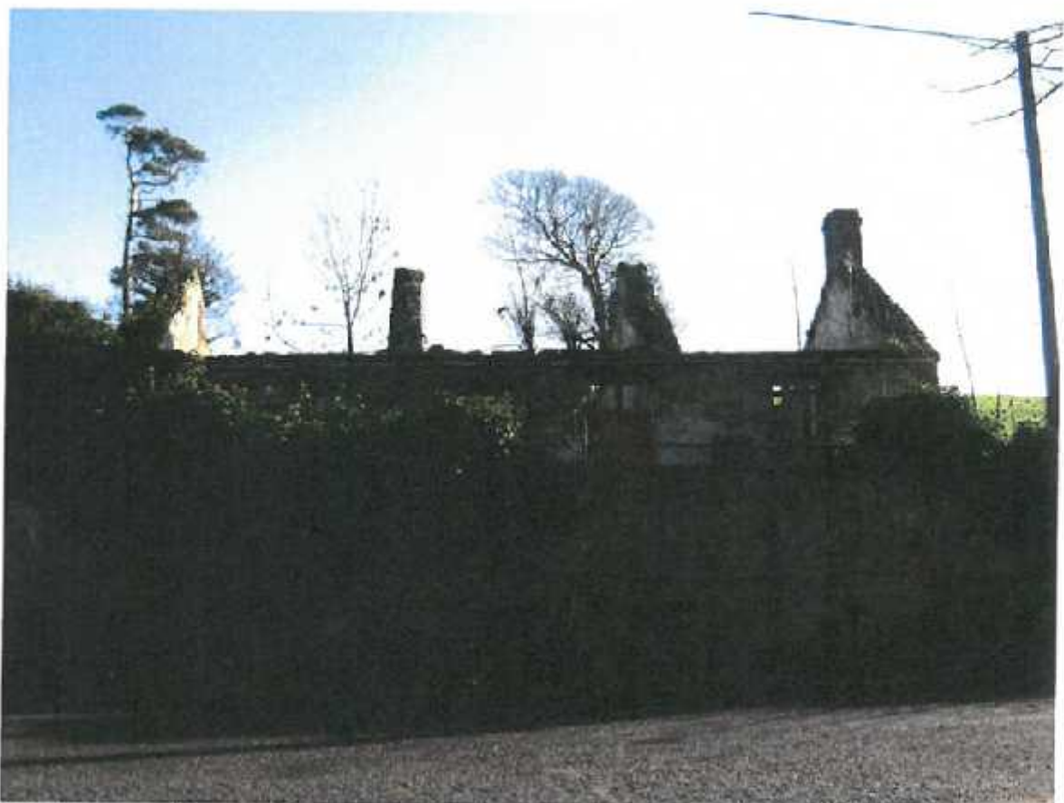
Existing Dwelling RHS Frontage to Viantown Road.
