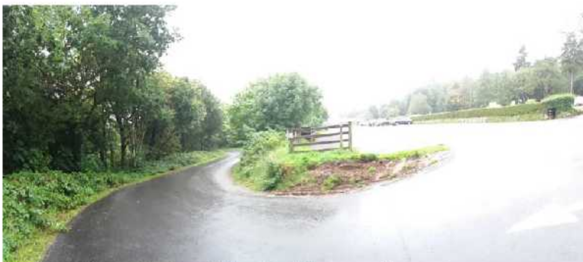
North of existing embankment (View of existing car parking area)
