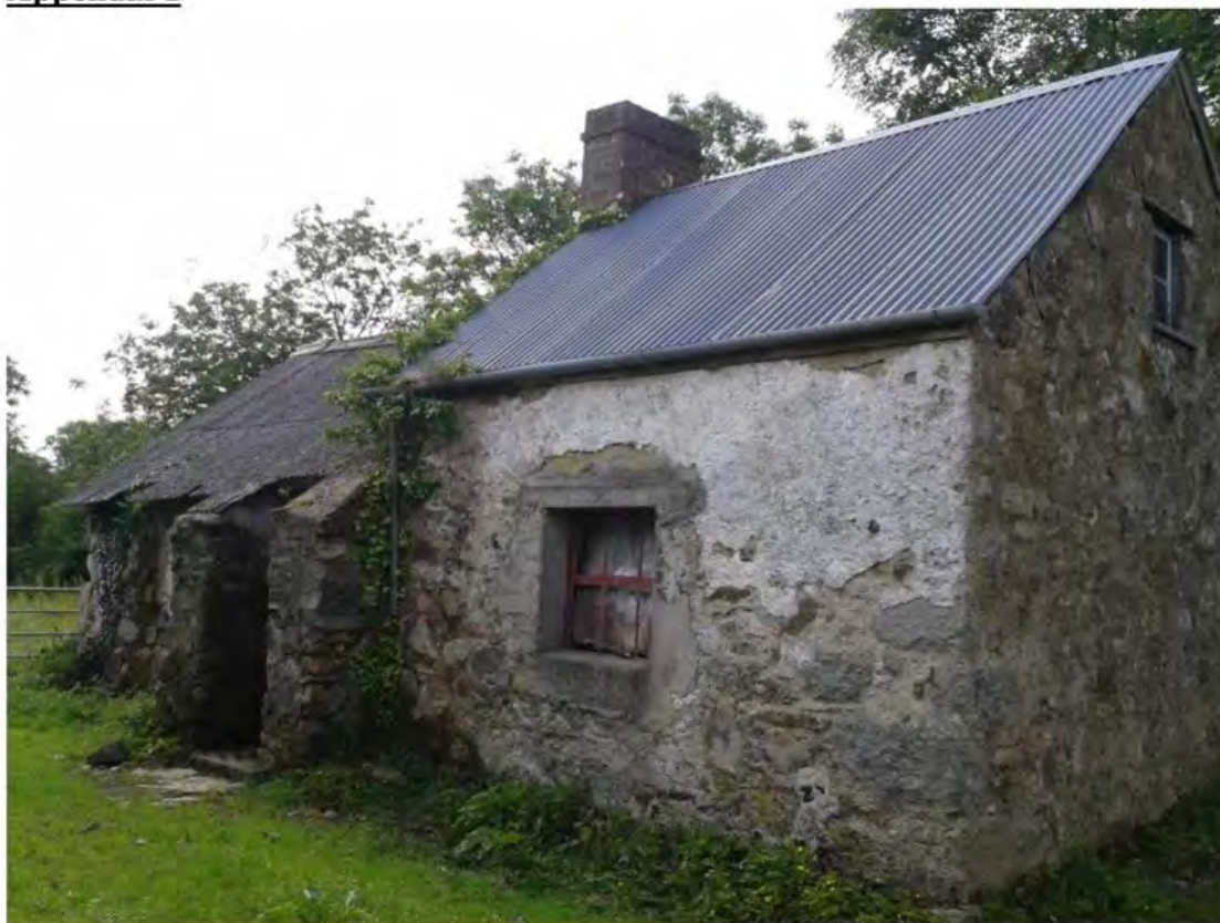
Photograph 8 – single building relating to planning approval P/2015/0050/F which was deemed to have satisfied the visual linkage test
