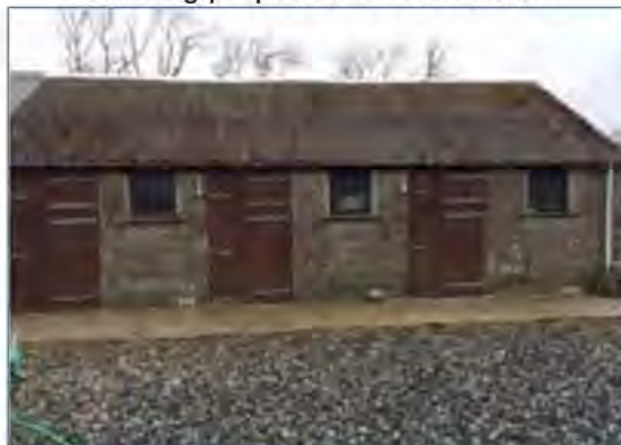
Building proposed for conversion
