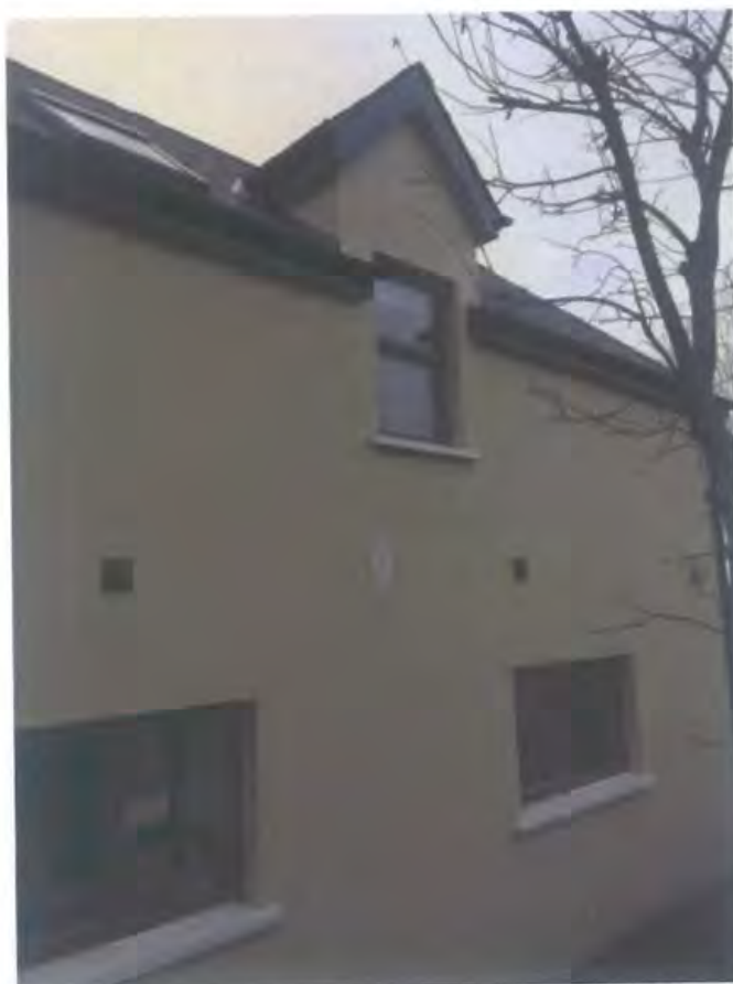
Existing Dormer Window.
