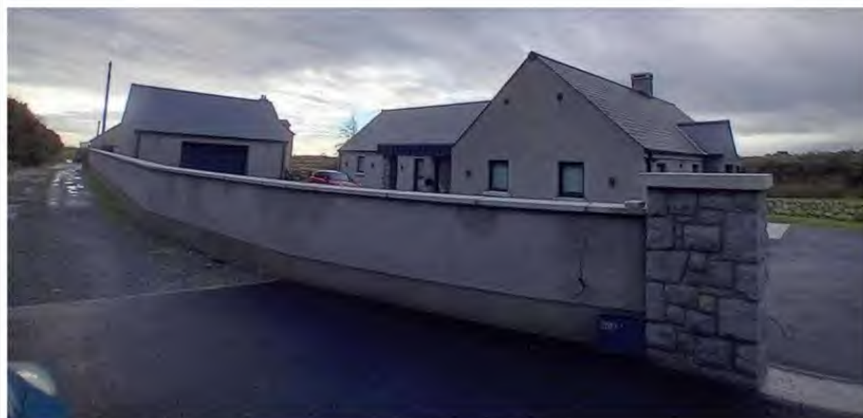
Figure 9 Photo of 90a and garage
