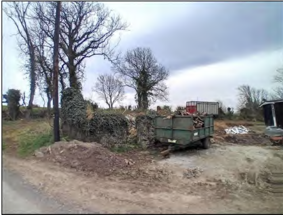
Figure 3- Southern and Western Elevations Intact
