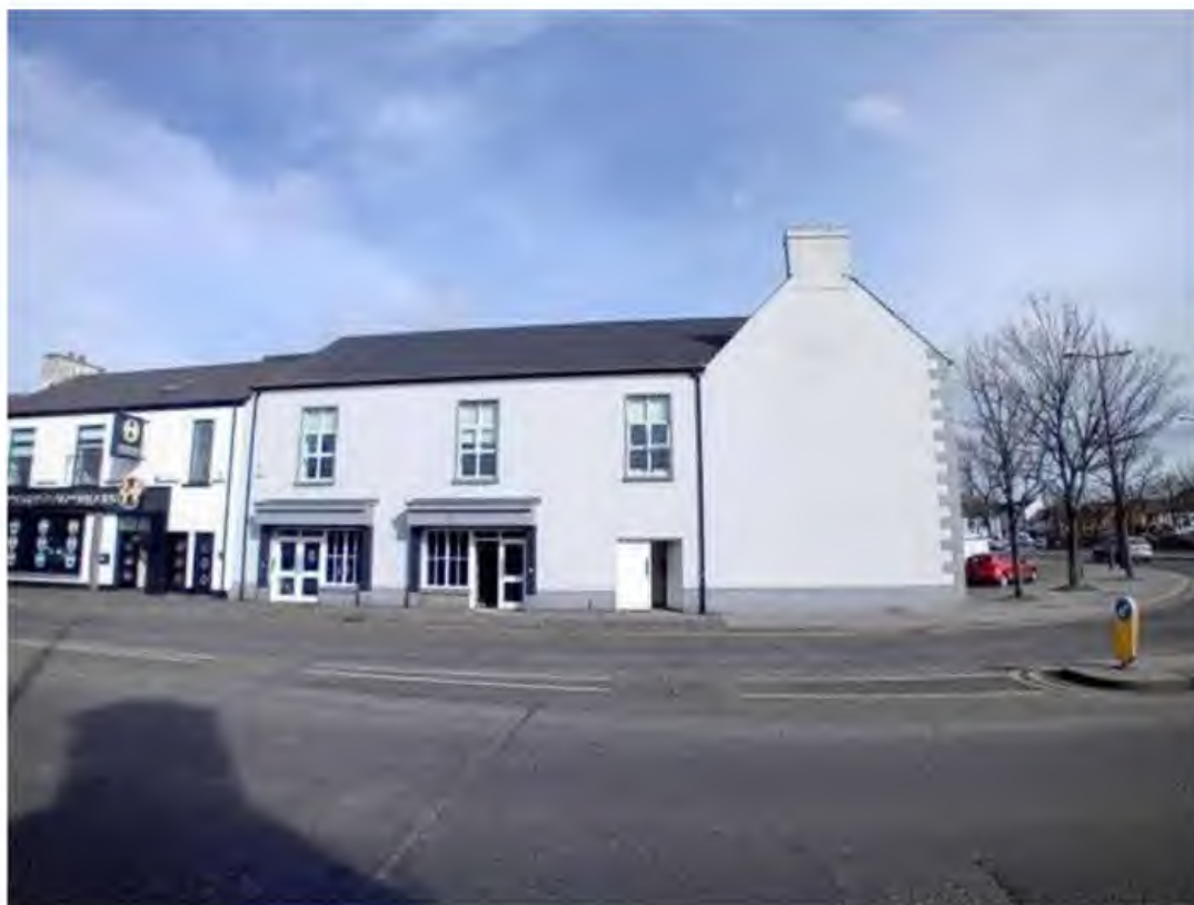
Figure 2- View of Application Site From Newry Street
