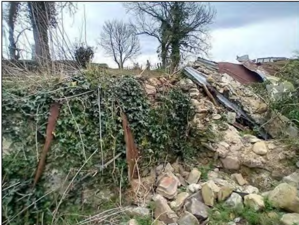
Figure 4- Northern elevation intact
