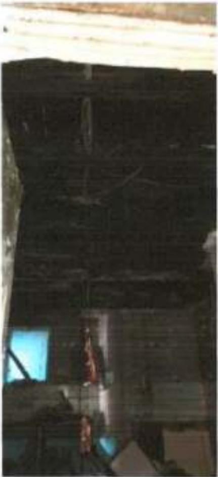
Image 5 – Second floor joists with significant rot and in complete disrepair
