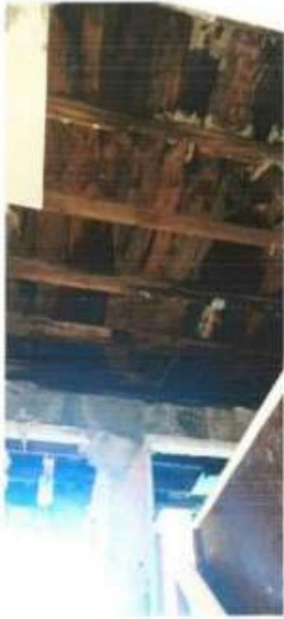
Image 6 – Second floor joists with significant rot and in complete disrepair
