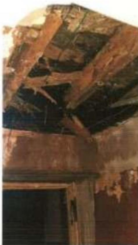
Image 4 – First floor joists with significant rot and in complete disrepair
