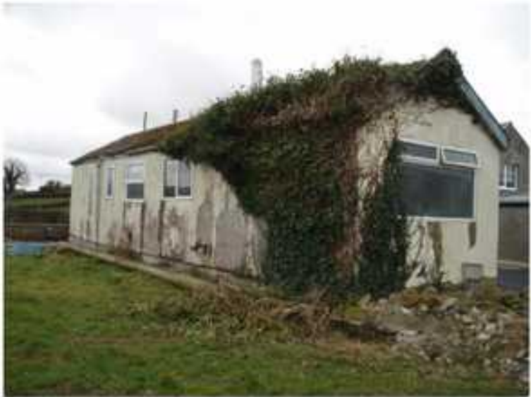
Side elevation of Structure
