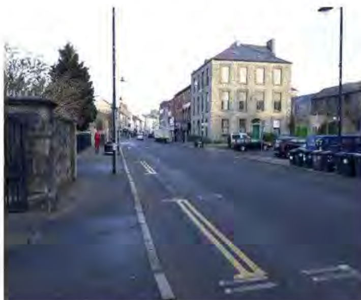
Existing paving on John Mitchell Place
