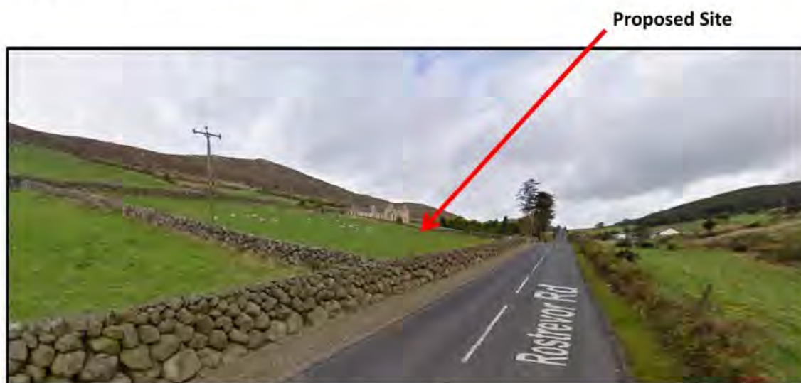
Image 1 - Goole Image of Application Site
