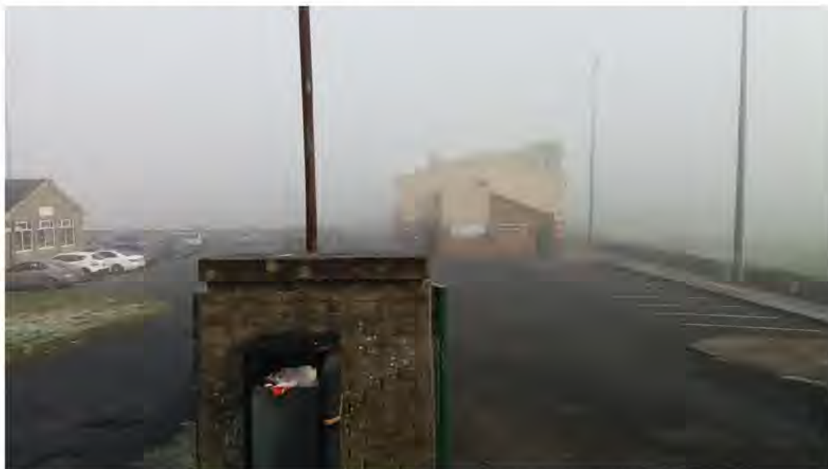
Above: existing St Mary's GAC Clubhouse
