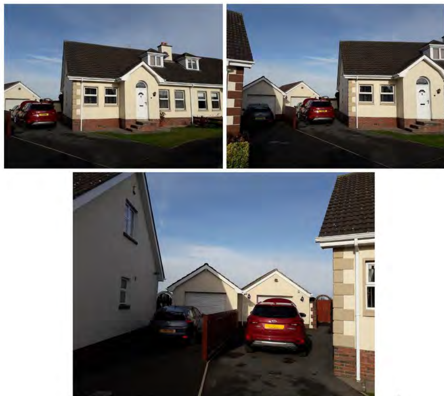
Front elevations of 6 Kinedale Cottages showing the existing detached garage
