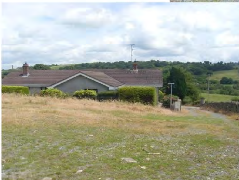
View towards No. 29a and Billys Road
