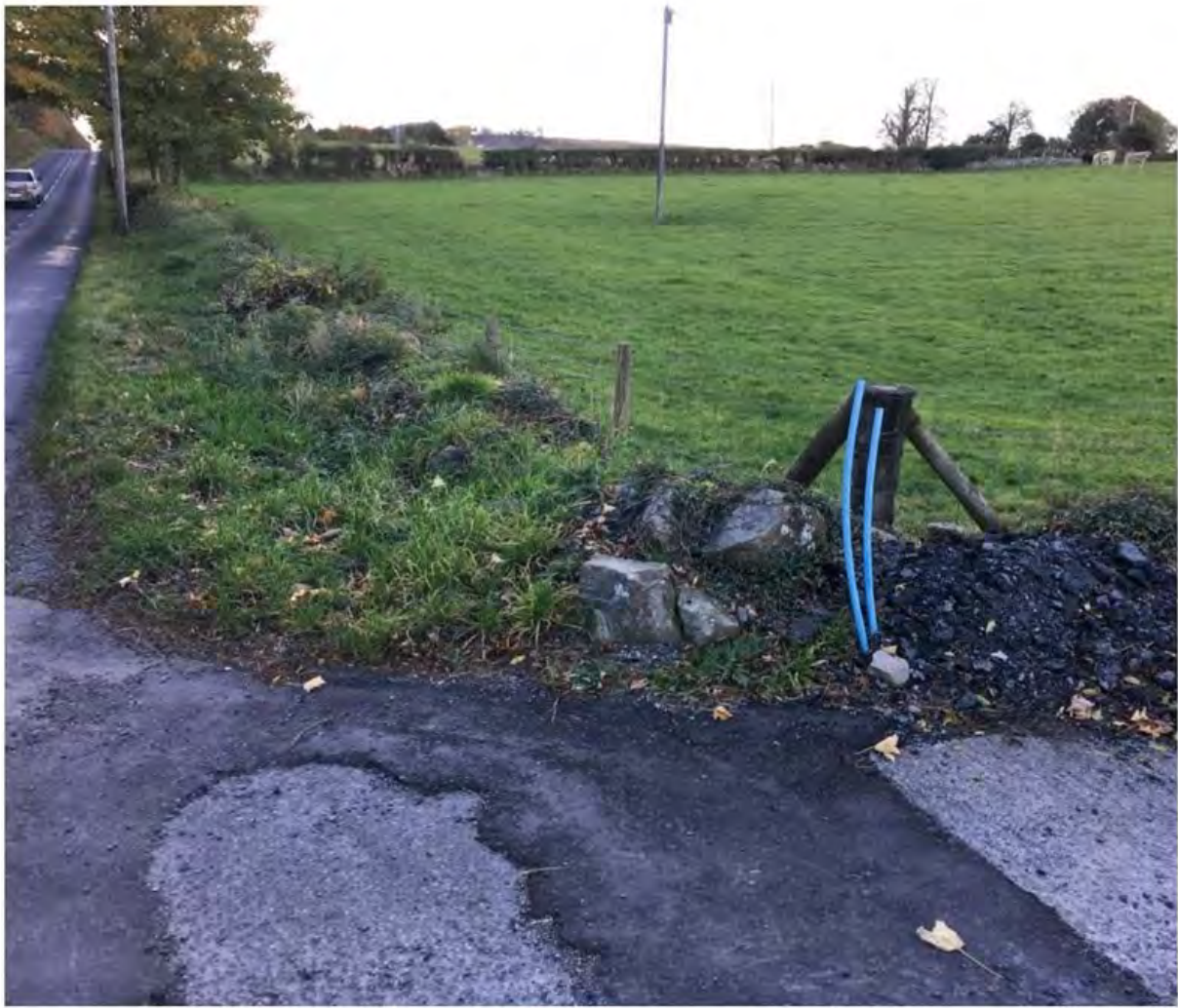
ACCESS ONTO THE HILLTOWN ROAD LOOKING TOWARDS HILLTOWN. THIS IS WHERE DELIVERY LORRIES HAVE TO PARK FOR UP TO 2 HOURS TO OFFLOAD. THERE ARE OBVIOUS HEALTH AND SAFETY ISSUES WITH THIS.
