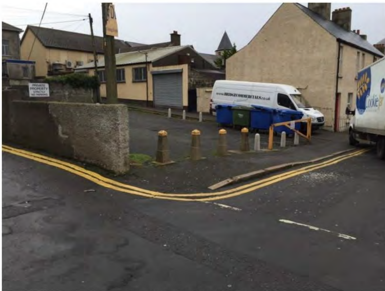
Photograph of the rear of the site.
