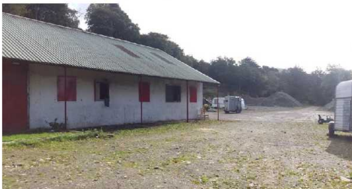
Upper part of site and existing building
