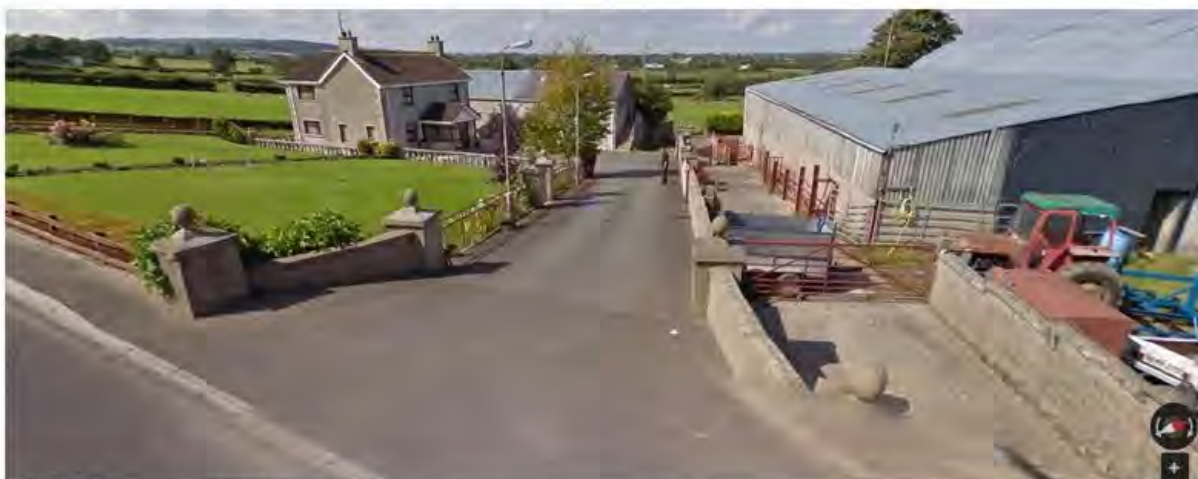
Existing access point 2 to No. 50
